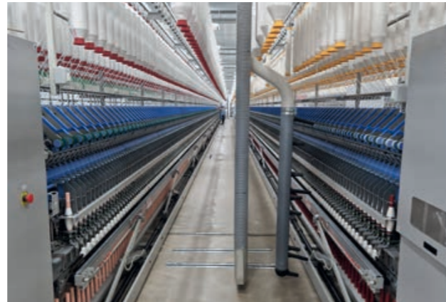
Figure 19 Clean surrounding conditions in ring spinning
