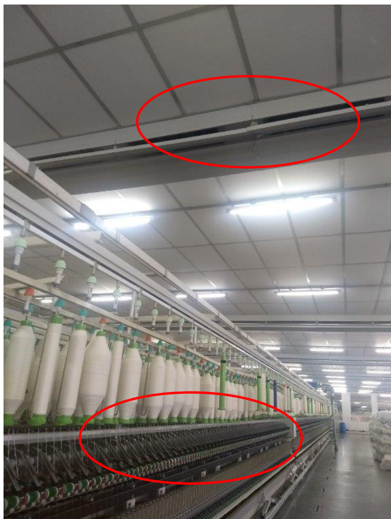
Fig. 5: Defective flap above the machine, causing dust and fluffy fiber bundles to fall on to the machine.
